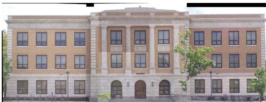
Figure 3. The façade after rectifying eight images
