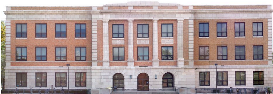
Figure 5. The façade's final rectified imagery subsequent to rescaling of the central part mosaic
