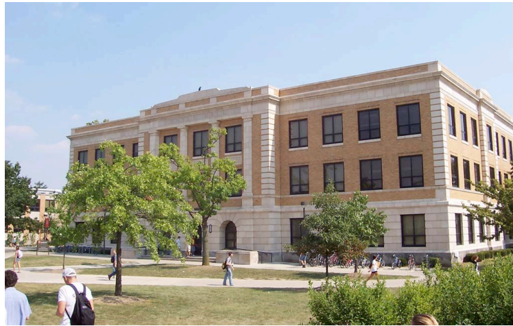
Figure 1. Hayes Hall: main façade looking west
